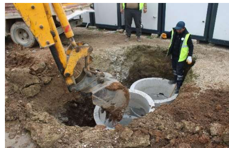
WASH team supervising septic tank installation in an ITS.
